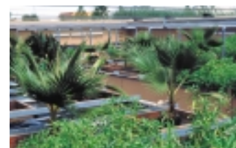
Open aerobic reactor.
